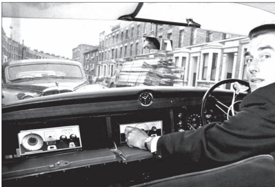
Fig. 2: The photograph was kindly sent to me by Ian Dilworth G3WRT. It shows the Codar AT5/T28 pair mounted in the 'cupboards' of (we believe) a Rover P4. Unfortunately, Ian can't remember where he got the photograph from. It would be very nice to find out who the gentleman was, and where the photograph was taken. And I wonder what antenna he used? Can anybody help out?
